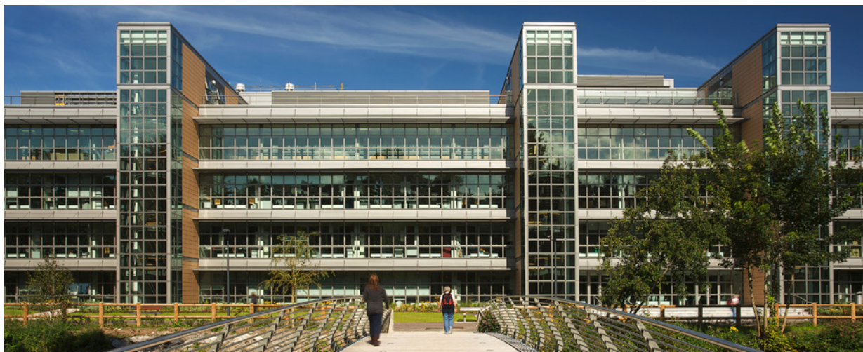
Western Gateway Building, University College Cork
